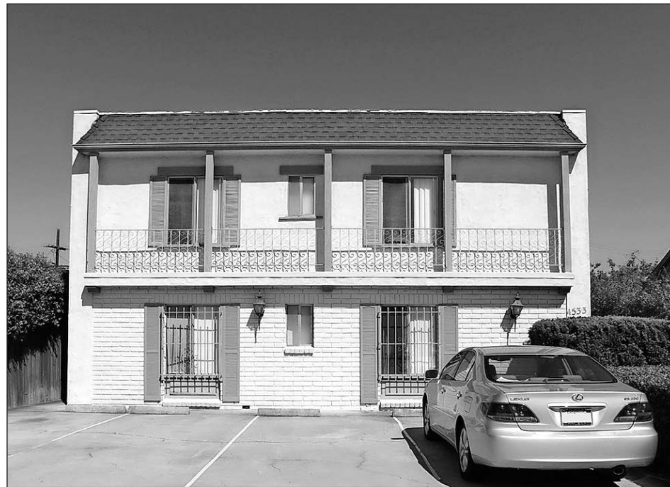
Photo courtesy of ACI Apartments
