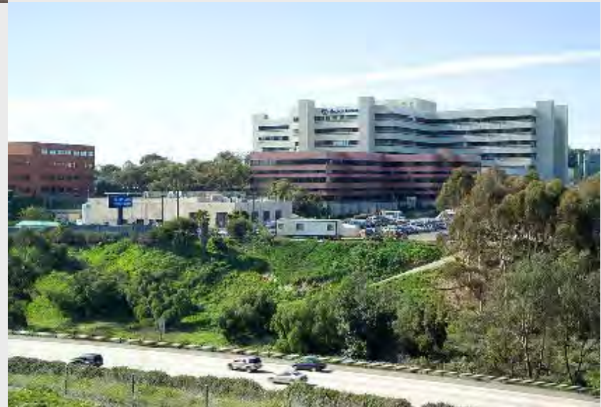
4.6 MW Mercury 50 San Diego VA Medical Center
