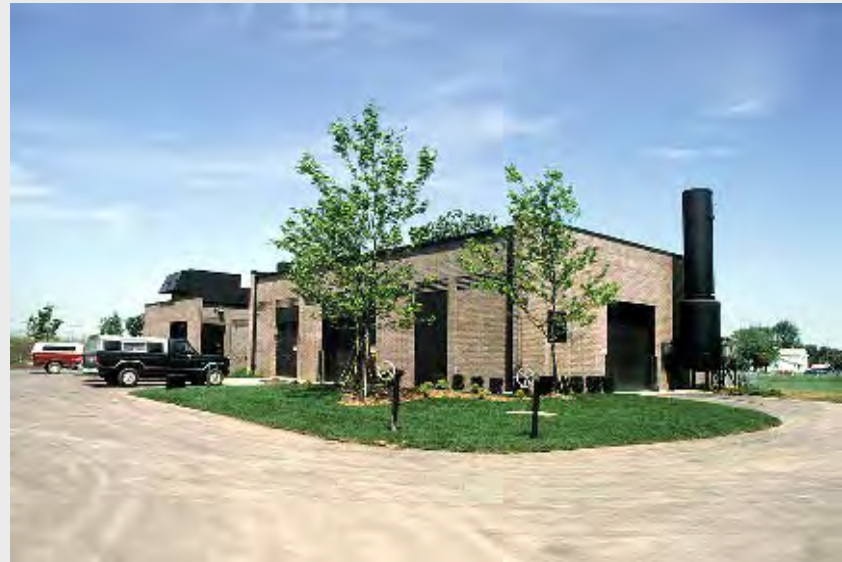
3.5 MW Centaur 40 Metro, Wisconsin Landfill
