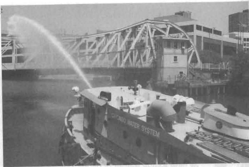
Figure 1. City workers hose down the Kinzie Street Bridge to prevent it from locking. Source: Chicago Sun-Times ; photographer: John White. Reprinted with special permission from the Chicago Sun-Times, Inc. © 2002.
