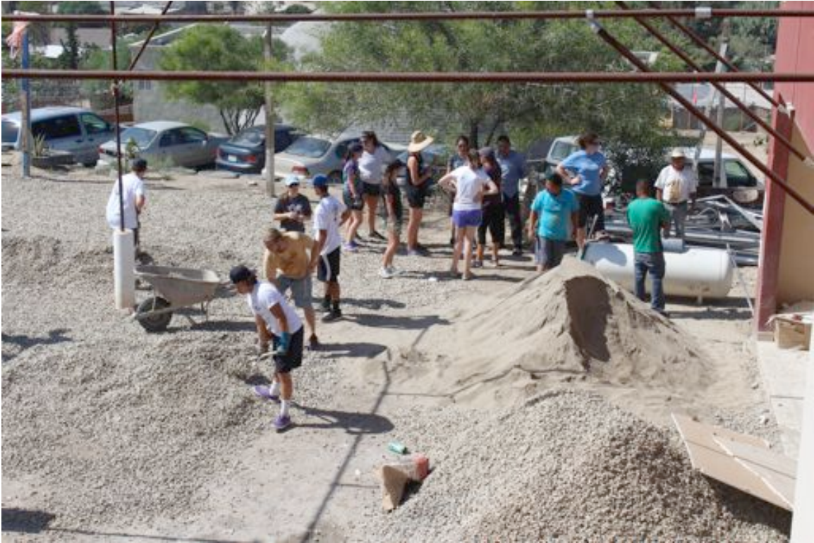
During the September Tijuana Day Trip, USD students helped with a renovation project for one of the chapels in Tijuana.
