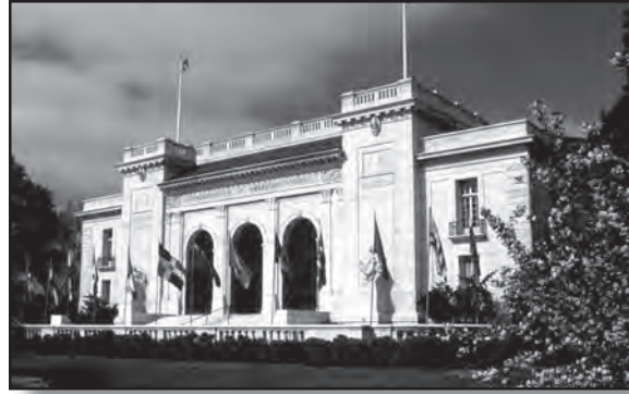
OAS Main Building (photograph provided courtesy of OAS)
