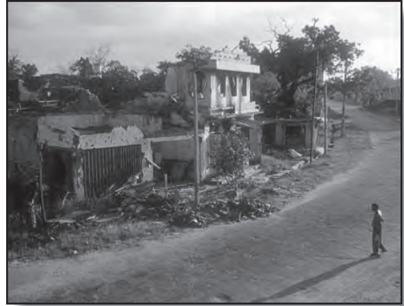
Destruction of civilian houses in Mannar
