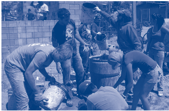
Participants in the Ibero Summer Seminar work with Esperanza build homes and schools of concrete and cinder blocks in Eastern Tijuana.
