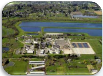
Waste Water Treatment Plant
