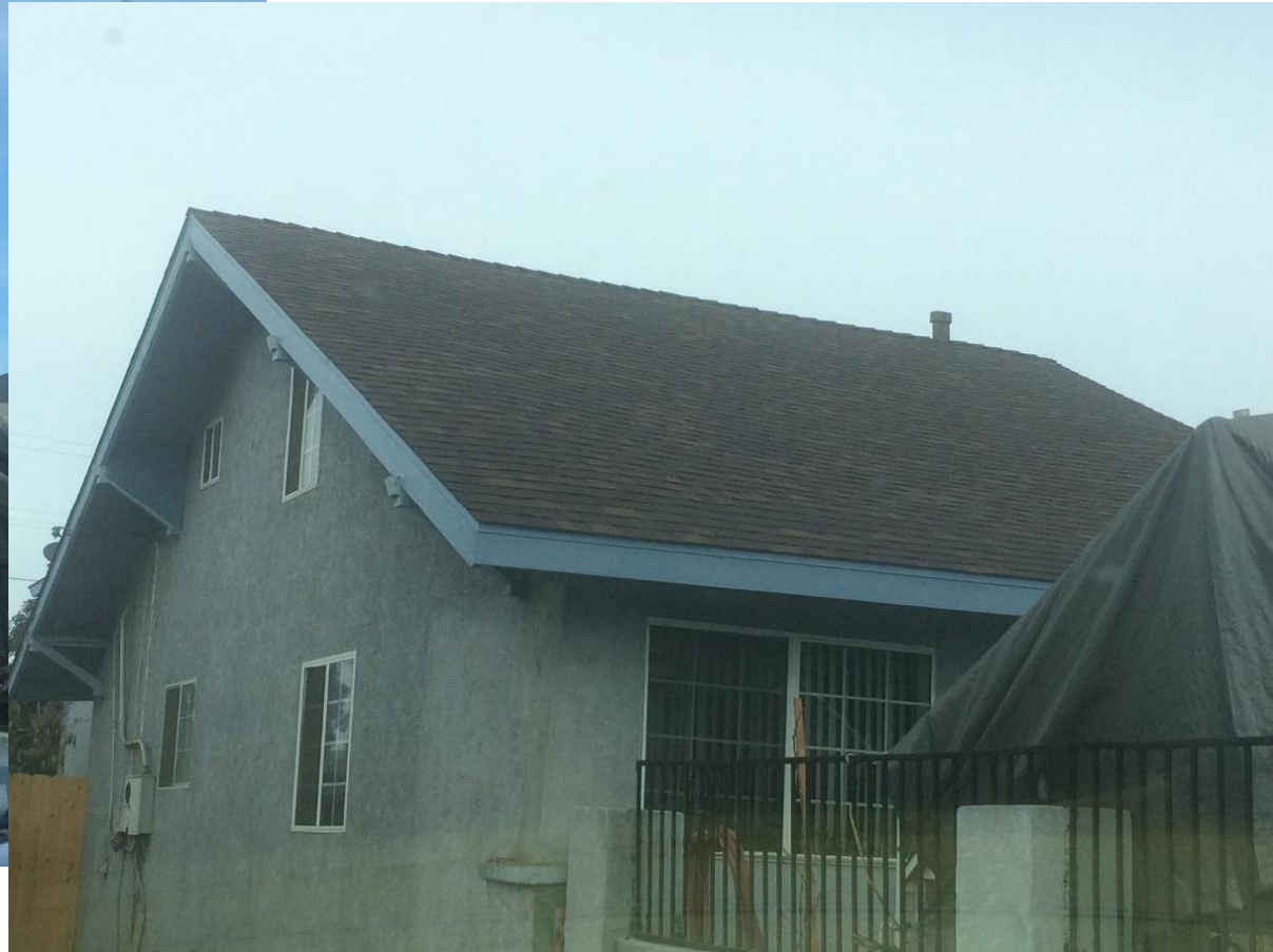
Left and Below: San Diego Habitat for Humanity Home Roof Rehabilitation
