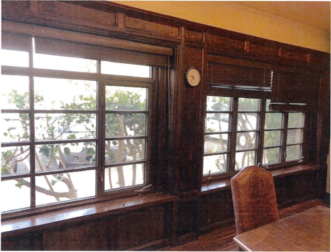
Wood Paneling Serra Hall
