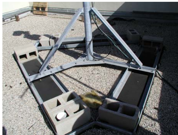
Figure 31: Stand on the Loma roof
