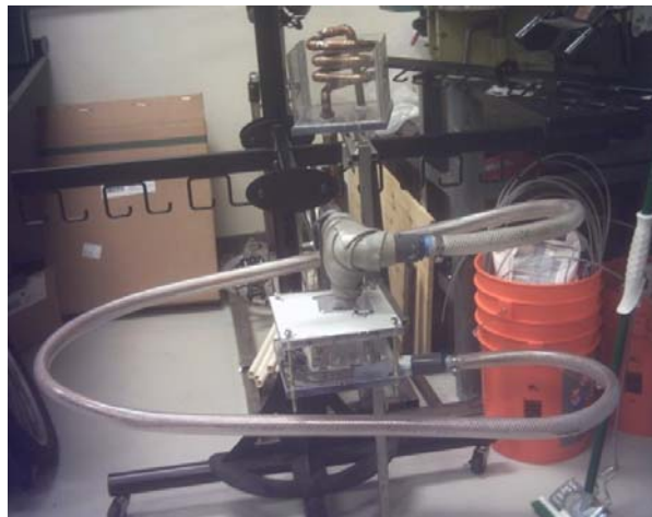
Figure 57: New heat exchanger
