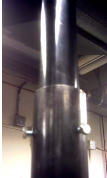
Figure 33: Telescoping pole joint
