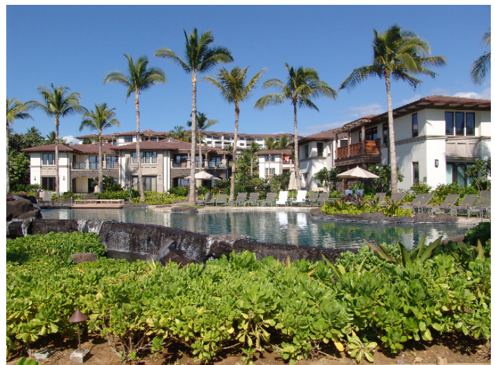
Phillip Thrash worked on this project: Wailea Beach Villas in Maui
