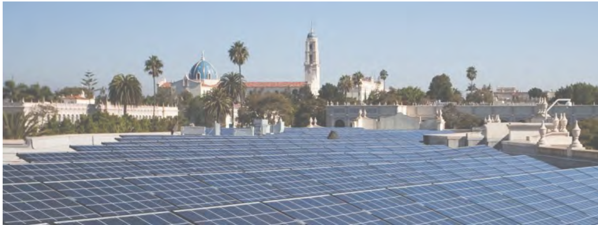
SOLAR PANELS POPULATE MANY ROOFS ON THE USD CAMPUS AND HELP THE UNIVERSITY POWER ITS FACILITIES
